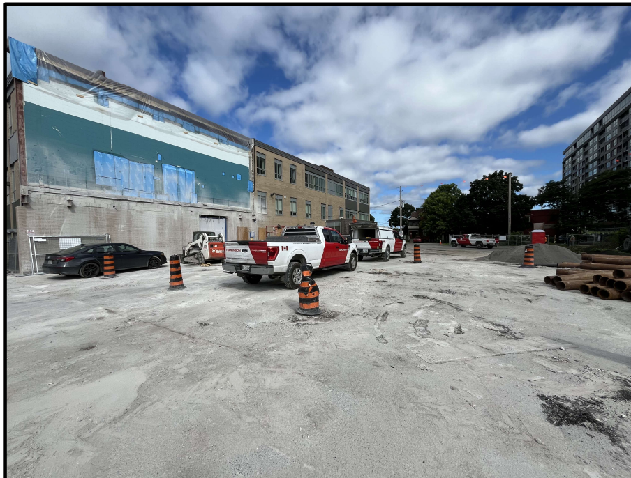
Preparation for Site Servicing
