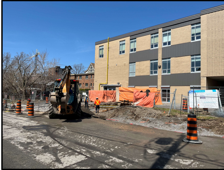
Utility Work on Arlington Ave
