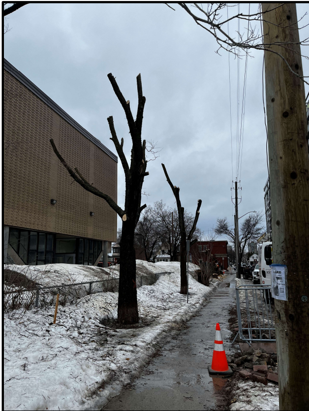
Removal of Existing Trees
