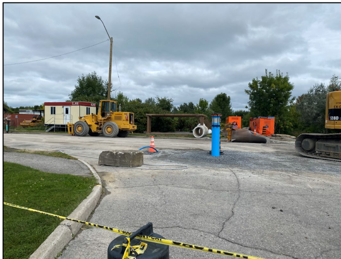
City of Ottawa Infrastructure Work at 302 Legget Dr
