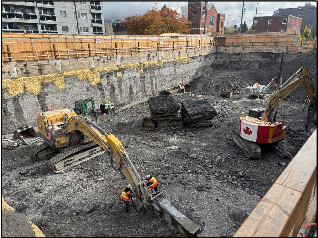
Construction Update – October 23, 2025
