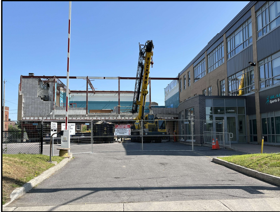
Demolition of Portion of Office Building
