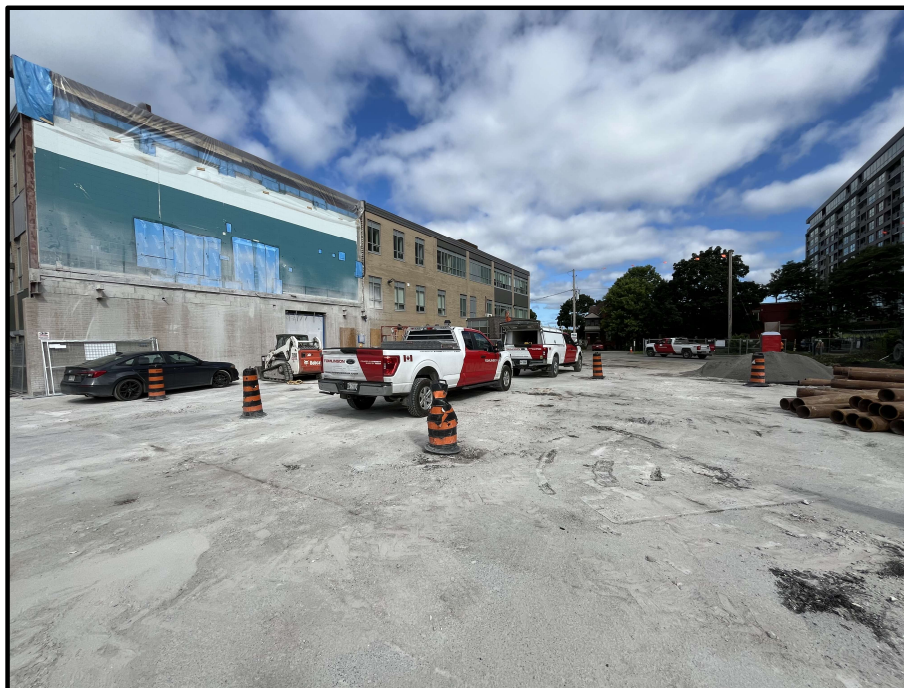
Preparation for Site Servicing
