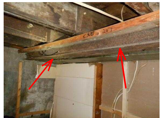
16. Beams: Steel I-Beam - Rusting and sagging was noted on older beam.
